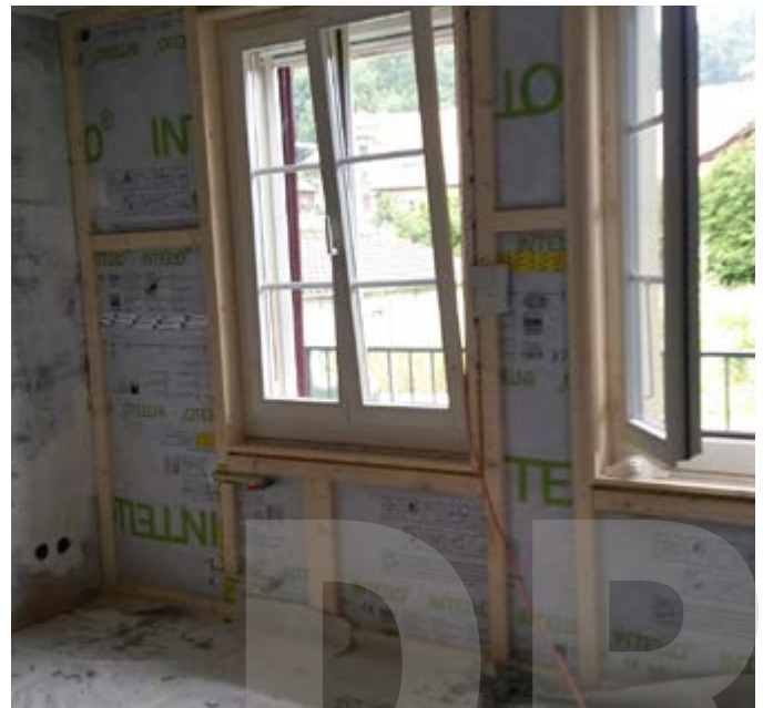
Figure 3.: Cellulose blow-in insulation on the inside of the wall (photo Auraplan)
