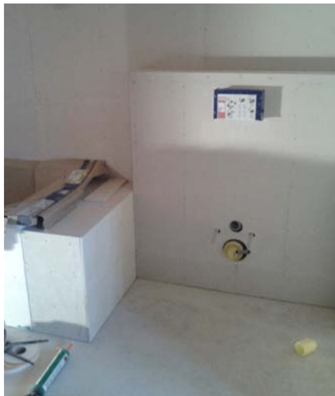
Figure 7: Fermacell planking in the bathroom (Photo Auraplan)
